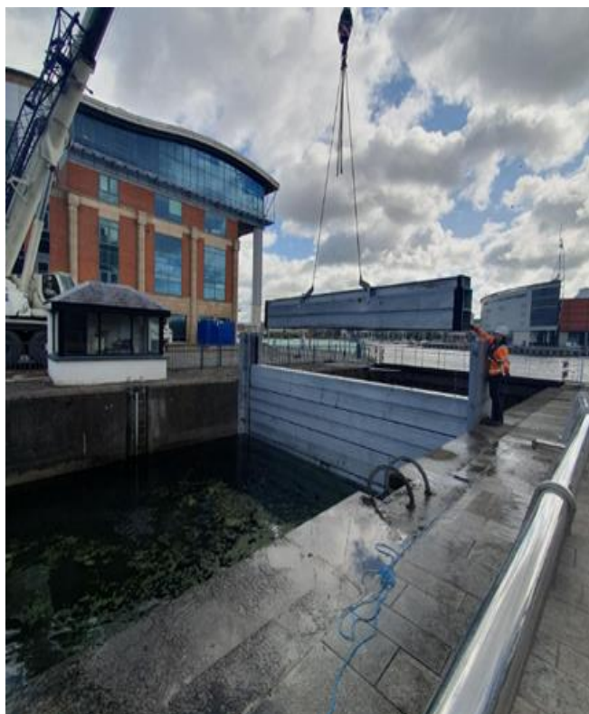
Stoplogs being deployed at Clarendon Dock August 2024 (DfI).
